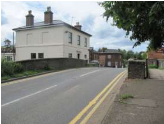
View along Hanbury Road looking north west at Bridge 44
