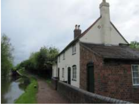
Lock keepers cottage, Stoke Pound
