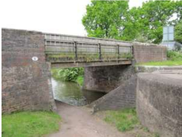
Bridge at Upper Gambolds
