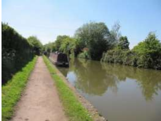
An enclosed section of the Canal
