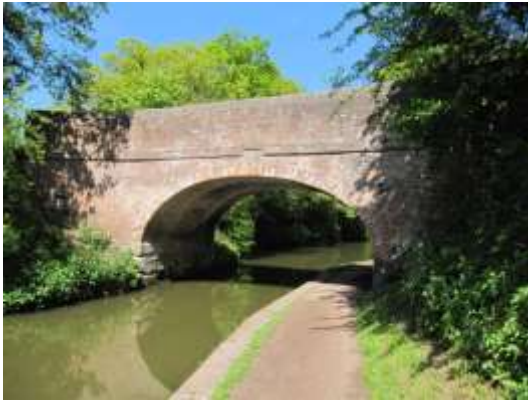
Typical Bridge, Bridge 55, with a concrete block number
