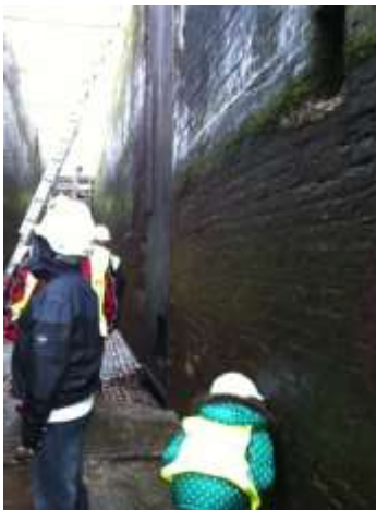
Lock 58, emptied for repairs
