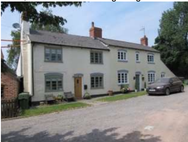
The Machine House to the right
