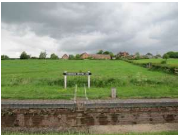
Bottom Lock in the Tardebigge Flight
