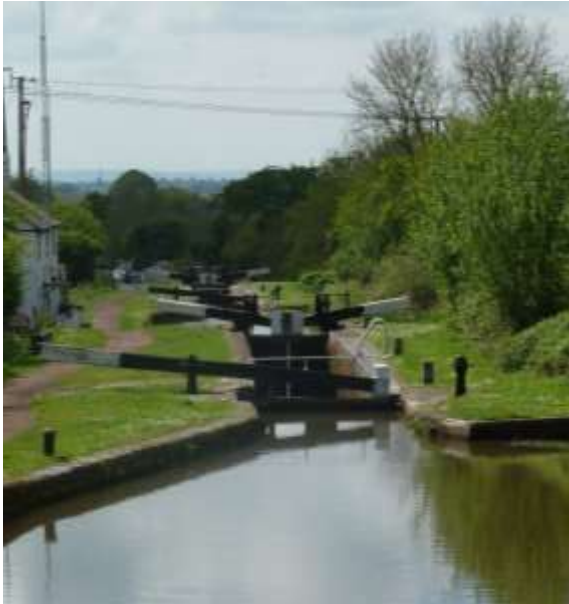
View from Lock 51, looking south west
