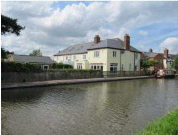
Properties along the Stoke Works stretch of the Canal
